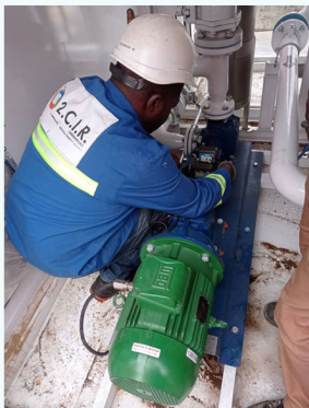
COMMISSIONING TRANSTANK LUBRICANTS
