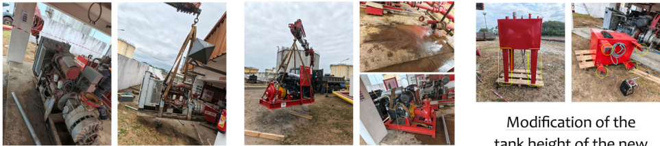
Removal of the old DCI motor-pump unit.
